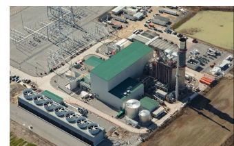
U.S. KEC Gas Combined Cycle Power Plant
