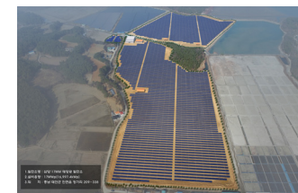
Samyang 17MW Solar Power
