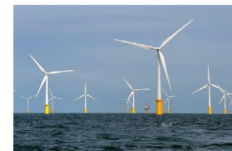
Jangbogo Offshore Wind Power
